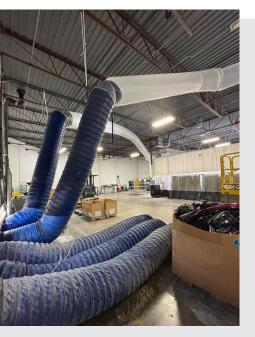
**Delivery Equipment and Meeting Needs -** A 25 ton air conditioning unit was ultimately selected to cool the areas of the facility, and a temporary generator was also required, given the limited power available. REIC was able to arrange for all the equipment, including the generator, along with delivery, setup and startup of the unit. Temporary ductwork was sent into the building, with flexible, temporary ducting spread throughout the interior to distribute cool air to areas needed most.
