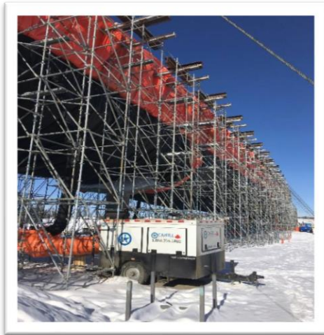
A CH15MS heater curing a large concrete section on a construction project
