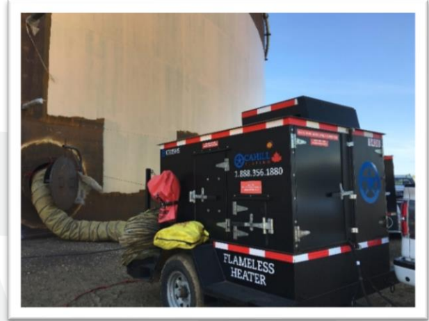
A single CH15HS heater providing hot, dry air to cure coating on a large tank evenly while keeping workers warm
