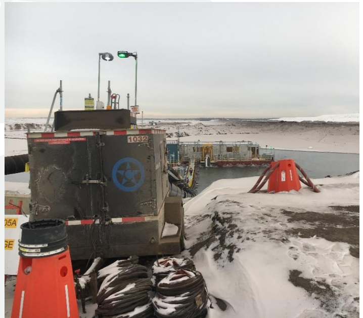
A CH15HS heater delivering hot air to a tailings barge from 500 feet away
